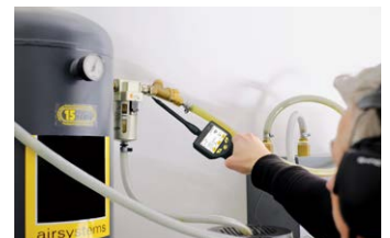
Leak detection with focus tube
